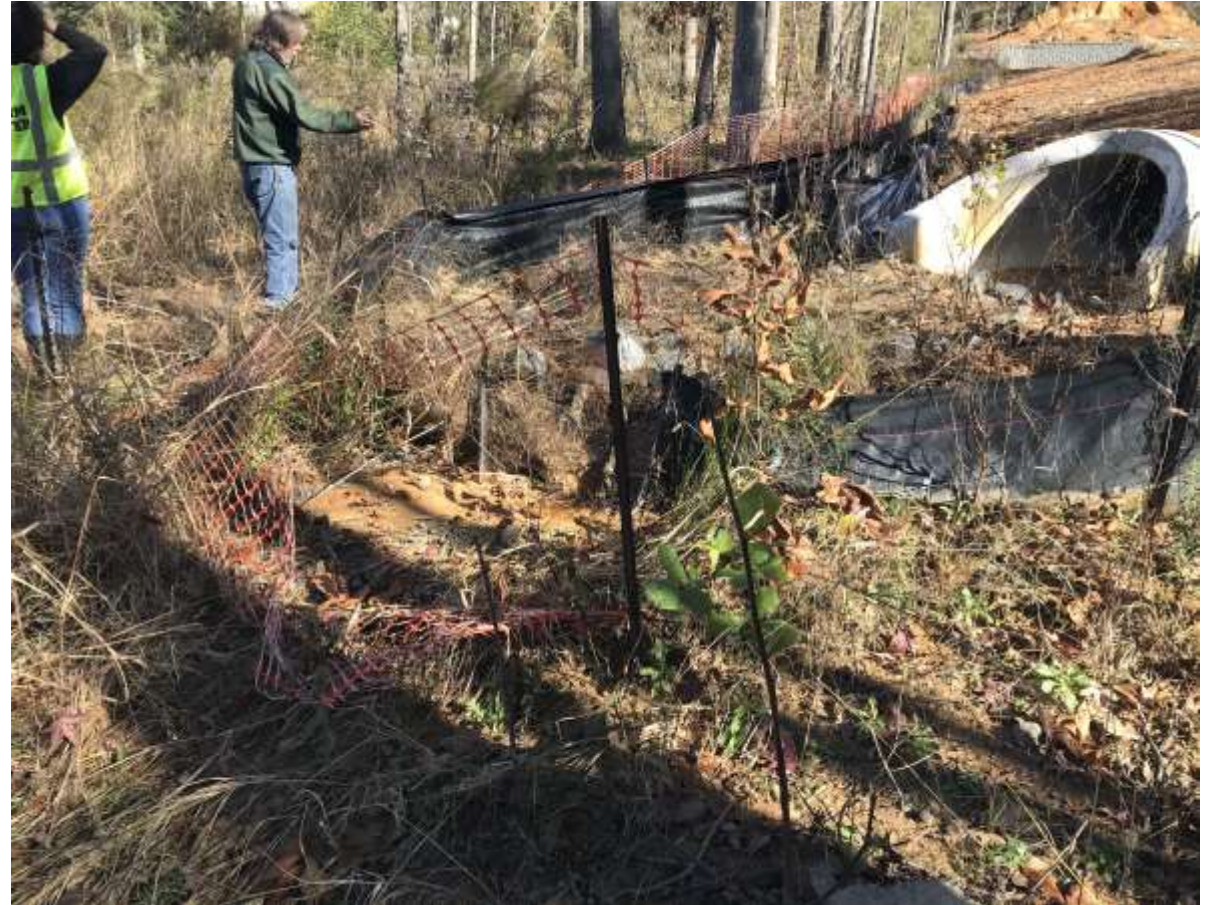
Stormwater outfall encroachment from a new development
