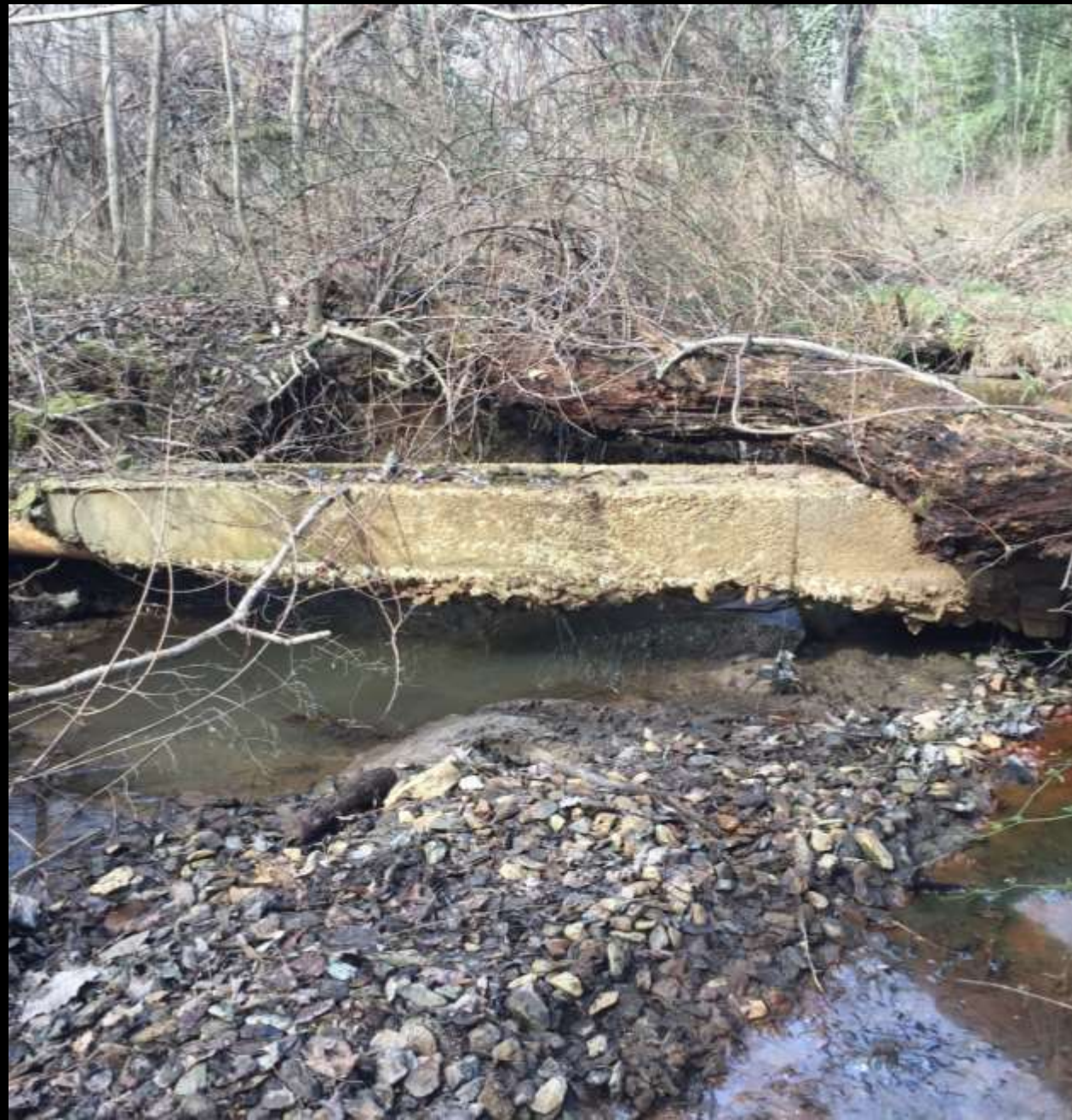
EXISTING CONDITIONS – EXPOSED SS AND UPSTREAM HEADCUTS
