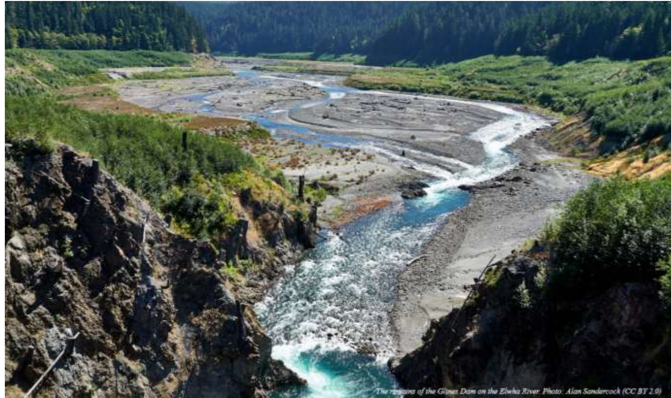
The remains of the Glines Dam on the Elwha River. Photo: Alan Sandarcock (CC BY 2.0)
