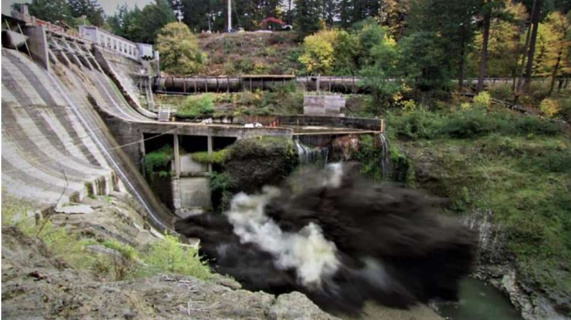
Condit Dam breached with dynamite on Oct. 26, 2011 (Andy Mazer, Oregon Public Broadcasting)
